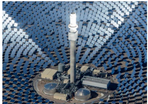
Figure 1: Solar Thermal power plant.
