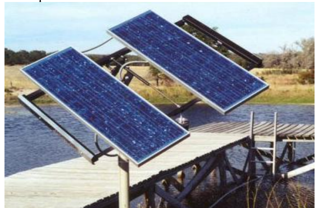
Figure 5: Zomeworks, Passive Tracker, UTRF-064.
