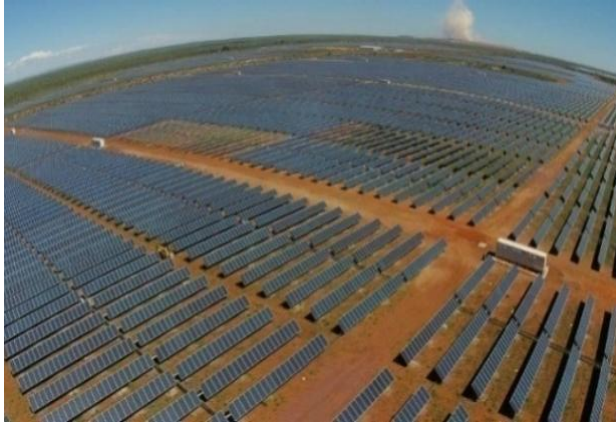
Figure 6: Atacama Photovoltaic (PV) solar plant, South America.
